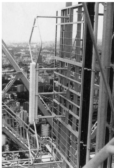
Fig. 10 A twin loop antenna with rectangular radiators.
