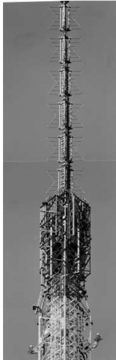
Fig. 4 The super-turnstile antenna on the top of the Tower.
